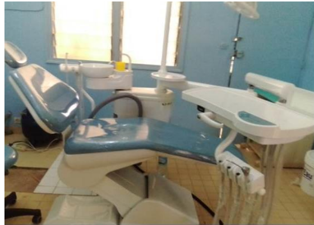
Figure 2 : installation equipment and wall painting
